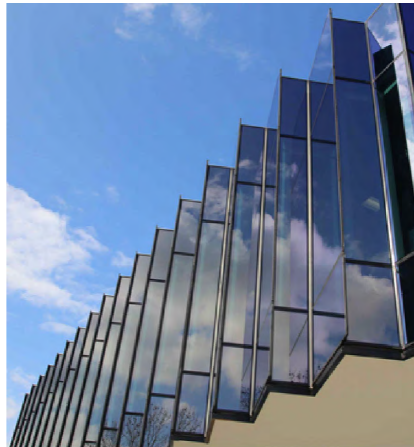
Springvale Cemetery, Clarence Reardon building. Internal & External corner mullions creating a zig zag effect
